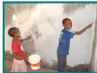
Mery and Calvin helping to paint the new classroom
